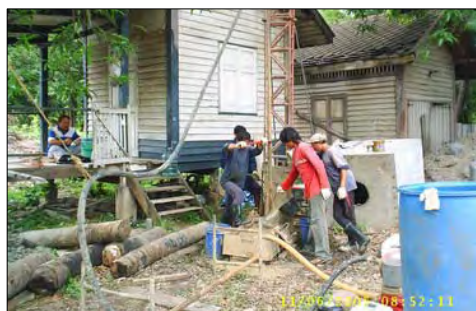
Soil Boring at Policy and Planning Office of Transportation
