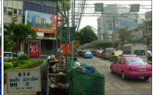
Soil Boring at Major Ratchayothin
