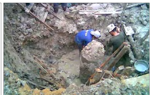
Bored Pile Head Preparation for Seismic Test
