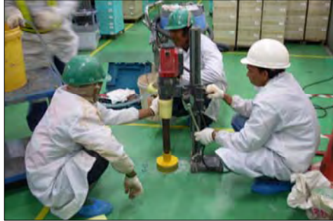
Concrete coring
