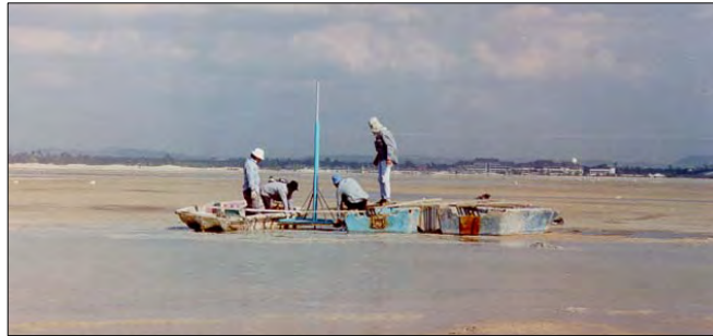
Surface Settlement Plate Installation
