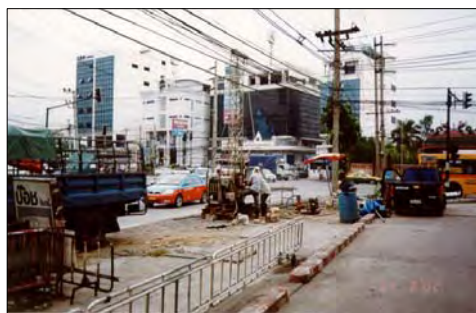
Soil Boring on at Poochao-Samingprai Road
