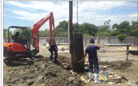
Dynamic Load Testing on Spun pile
