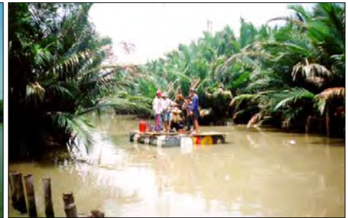
Soil Boring in Canal
