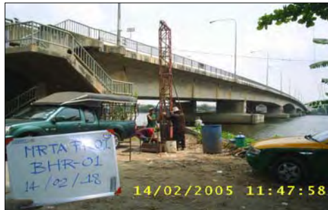
Soil Boring at Phra Nang Klao Bridge
