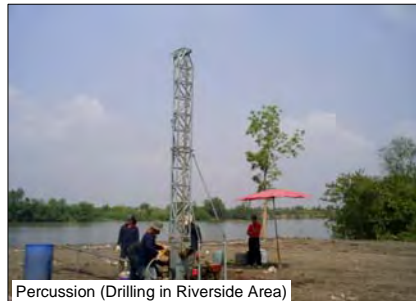
Percussion (Drilling in Riverside Area)
