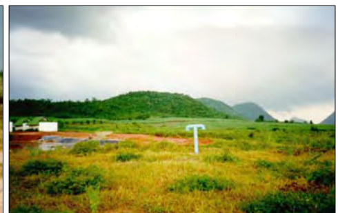
New Cell (Left) and Vent for a Closed Cell (Center)
