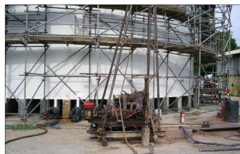
Soil Boring near the Existing Tank
