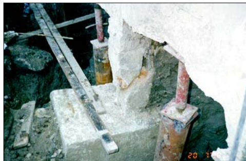
Investigation Settlement Causing Cracks in House
