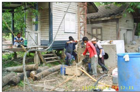
Soil Boring at Policy and Planning Office of Transportation
