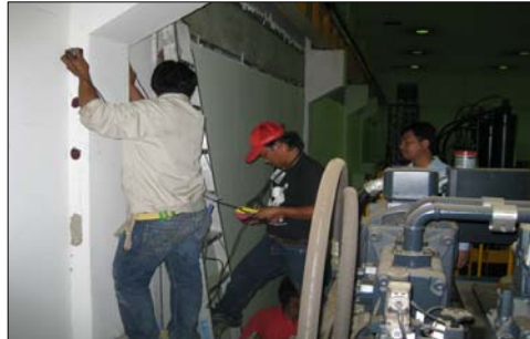
UPV Test at Column
