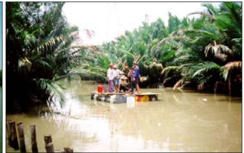
Soil Boring in Canal
