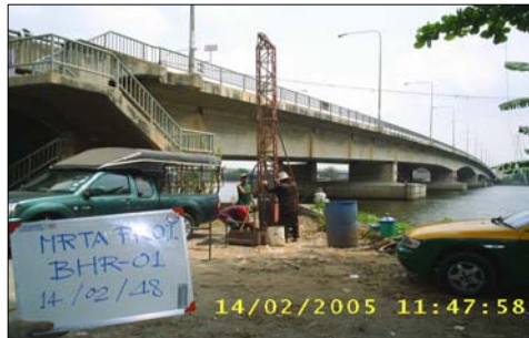
Soil Boring at Phra Nang Klao Bridge
