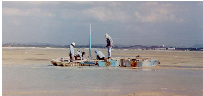
Surface Settlement Plate Installation
