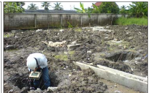
Seismic Testing on Driven Pile
