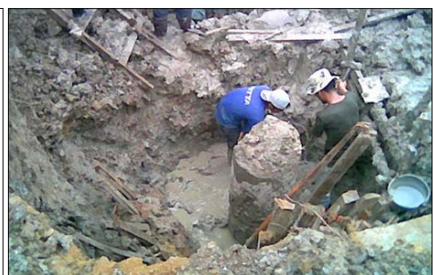
Bored Pile Head Preparation for Seismic Test
