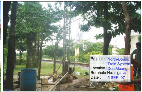
Soil Boring at Don Muang
